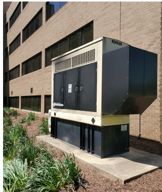
This is an example of a compliant remote stop (left) and backup generator at an ambulatory surgery center.
