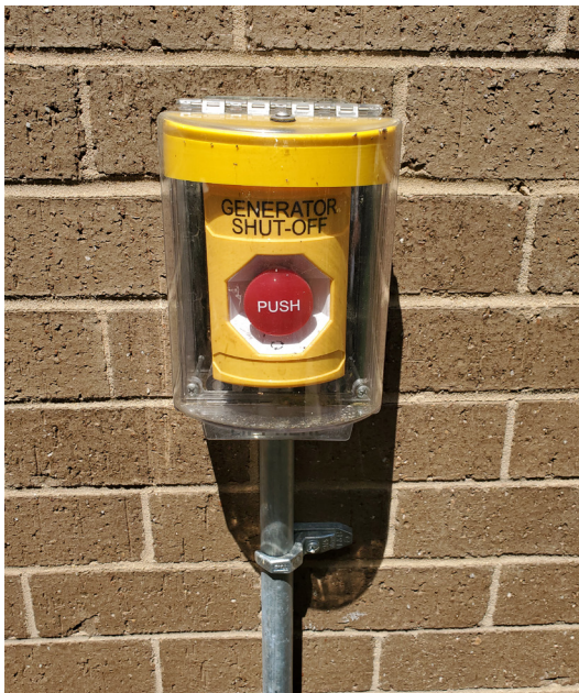
This is an example of a compliant remote stop (left) and backup generator at an ambulatory surgery center.
