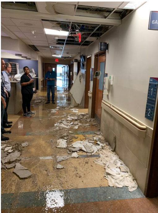
The devastating flooding required the gutting and rebuilding of Grady Memorial Hospital from the sixth floor down. PHOTOS COURTESY OF GRADY HEALTH SYSTEM. USED WITH PERMISSION.
